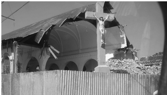
Figure 1. A church in Port-au-Prince, Haiti, after the earthquake.
